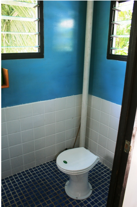
Figure 12: Waterless eco-sanitation toilet installed by the project
