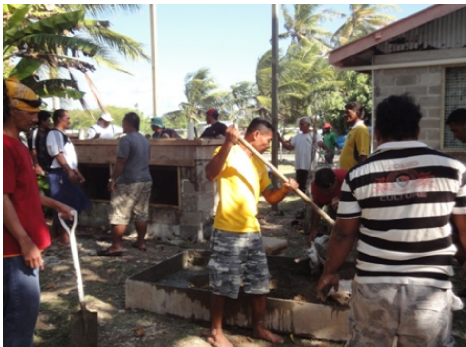
Figure 3: Construction workshop, convened for island construction workers to understand the principals of twin chambers and construct the toilets themselves
