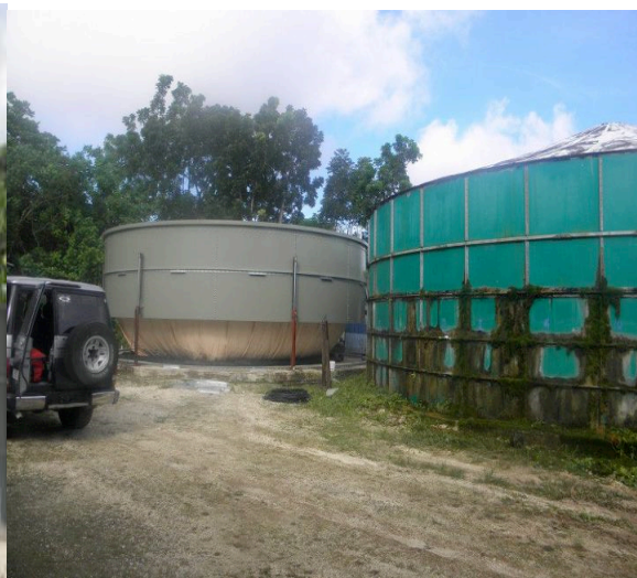
Figure 10: The new storage tanks (left) are located next to the old leaking storage (right) which had 456 kL capacity.
