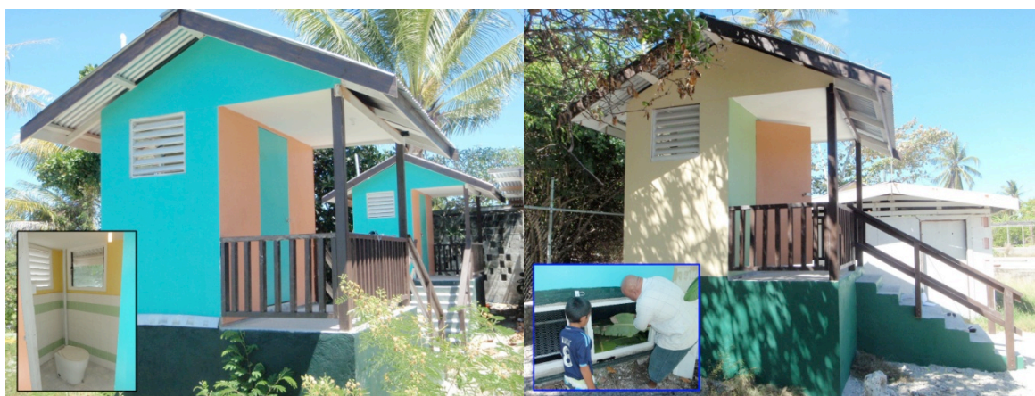
Figure 6 Prototype #3: Composting Toilets introduced to Schools at Kayser College and Anetan Infant School. The looks, odour (less), low maintenance, water saving and environment friendly are Communities key concerns.
