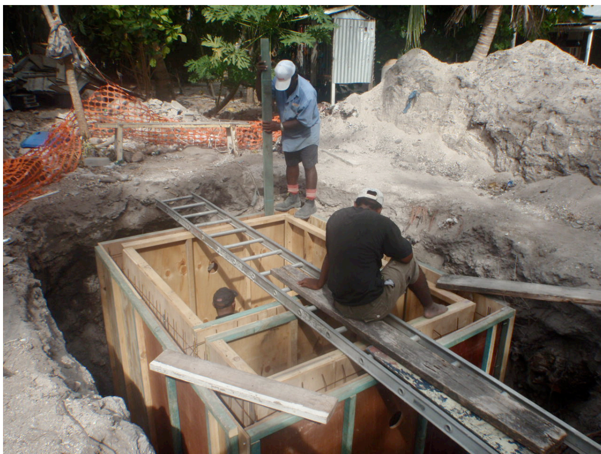
Figure 5 Contractor positioning the conventional Septic Tank mold at the demonstration community in Ewa. 22/02/2011.
