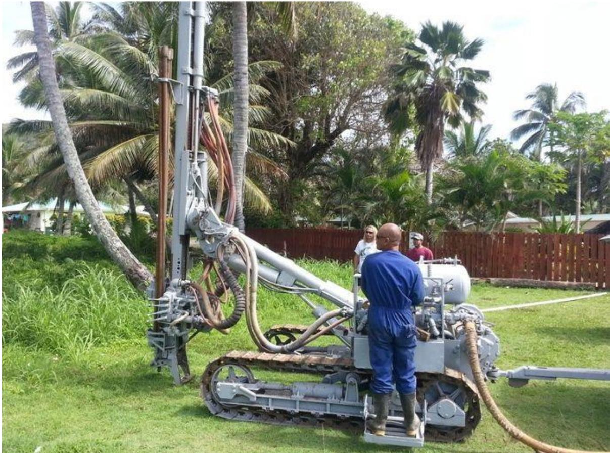
**Figure 9:** Drilling groundwater monitoring wells in the demonstration project area
