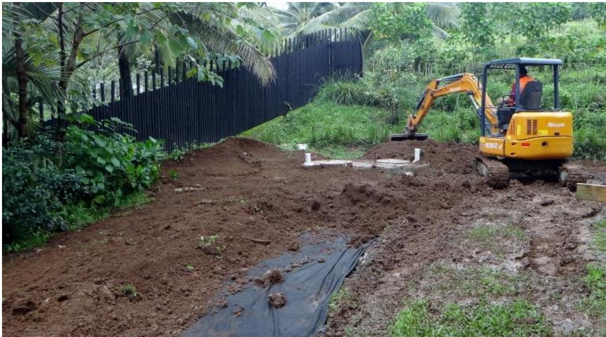
**Figure 7:** Package secondary treatment plant and land application system being installed at homes in the Muri-Avana area
