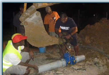
FSM consultant assisting the PWW Team with PRV installation
