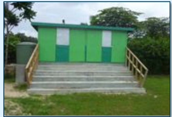
Composting toilet in Solway
