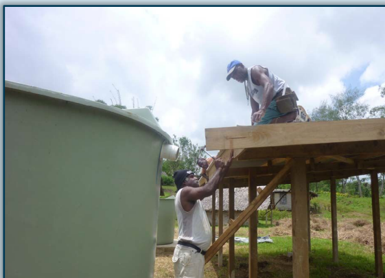
Construction of rainwater catchment at Butmas Community
