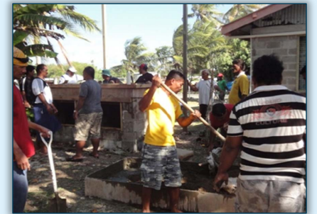
Falevatie construction workshop
