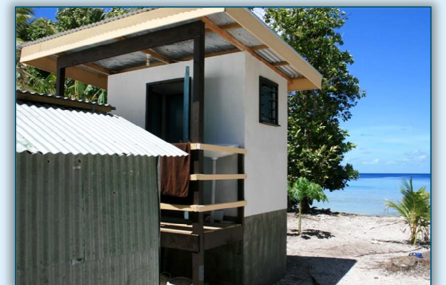
Installed composting toilet "Falevatie"
