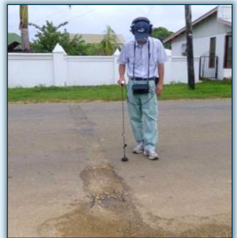
Leak detection in Neiafu
