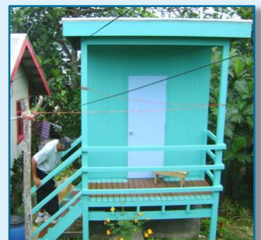
Composting toilet in Fungamisi
