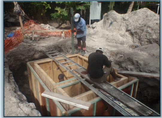
Contractor positioning the conventional septic tank mould in Ewa
