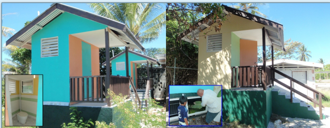
Composting toilets introduced at Kayser College and Anetan Infant School; addressing community concerns of odor, appearance, water efficiency and easy maintenance
