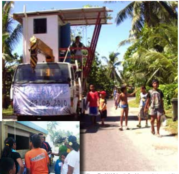
Above: The 2010 Falevatie Roadshow was instrumental in changing negative perceptions about compost toilets.
