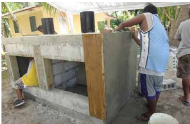
Above: Local builders constructing a compost toilet at Laura Village, RMI
