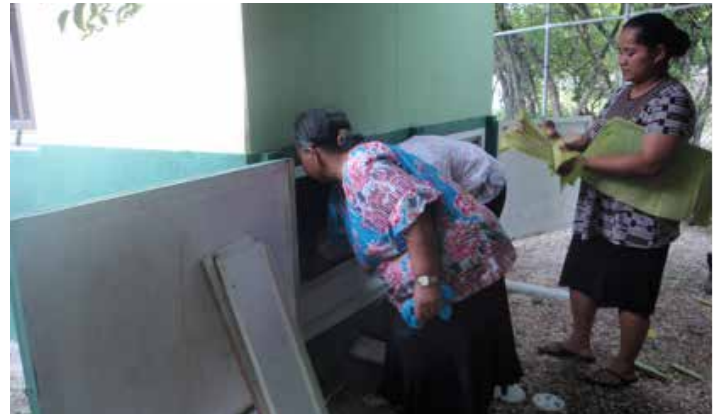
Teachers at Ewa School inspecting the compost toilet and learning how to maintain it
