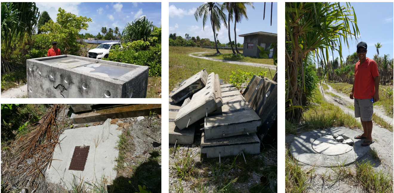
Figure. 2: Design of wells or bore holes at Bonriki/Buota Water Reserve (Photo: S. Sauni, 2019)
