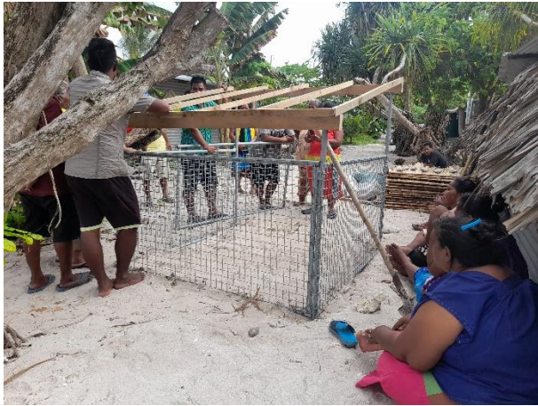
Figure 4. Pigpen completed with roofing left
