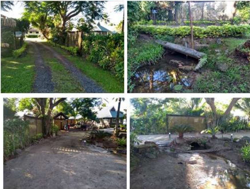
Muri Beachcomber/Night Market existing culvert
