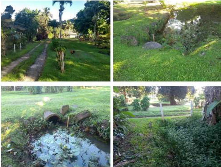
Aqua Café Access existing culvert
