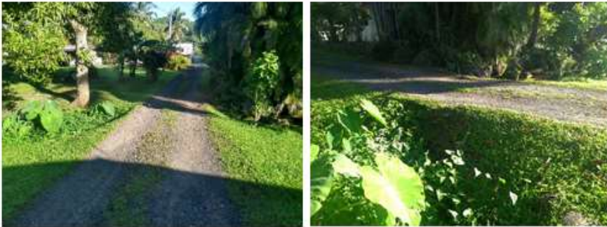
Access Opposite Te Ara Museum existing culvert
