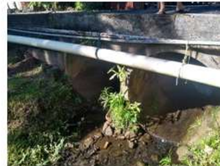
Flame Tree Villas access road existing culvert
