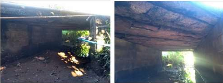
Access north of Pacific Resort existing culvert
