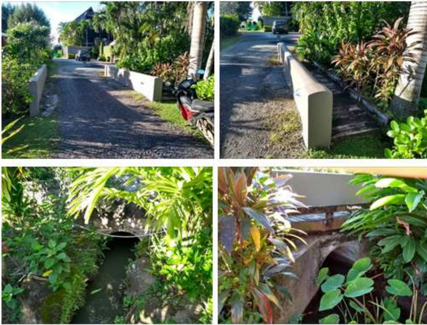
Te Vakarua existing culvert
