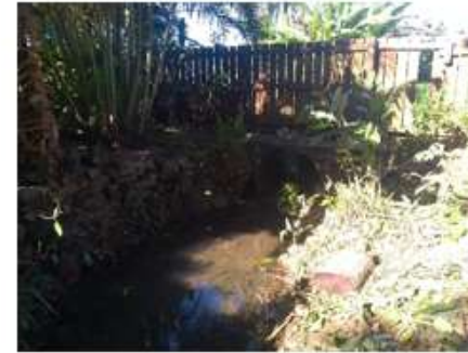
Existing culvert at boundary with rugby field
