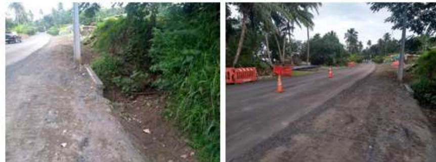
Existing Ara Tapu cross culvert south of Avana Bridge
