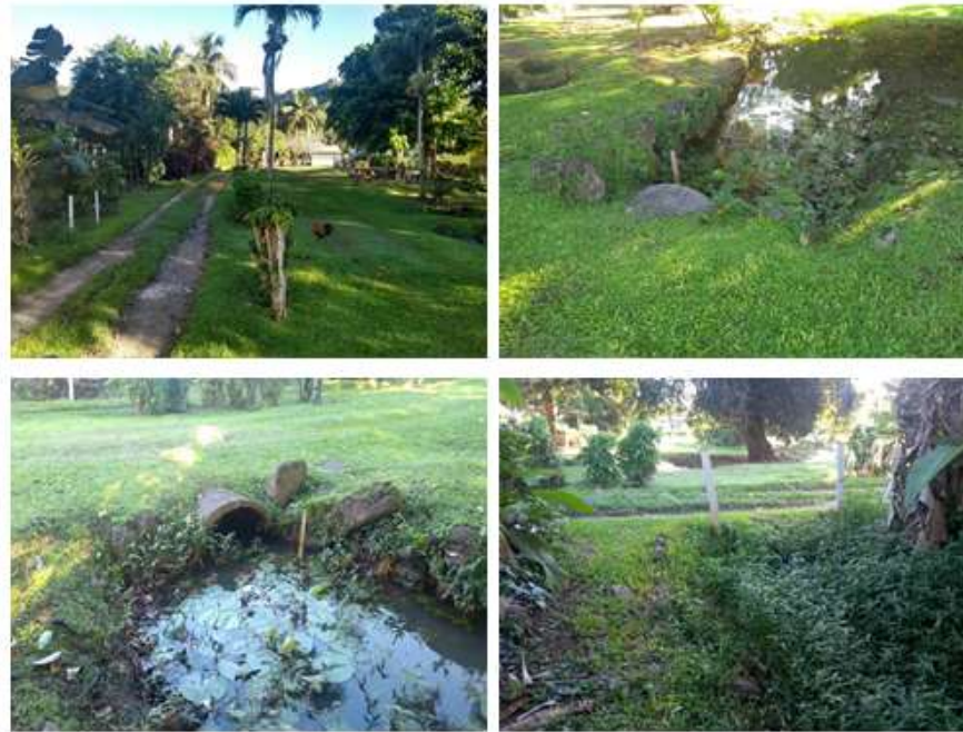
Aqua Café Access existing culvert
