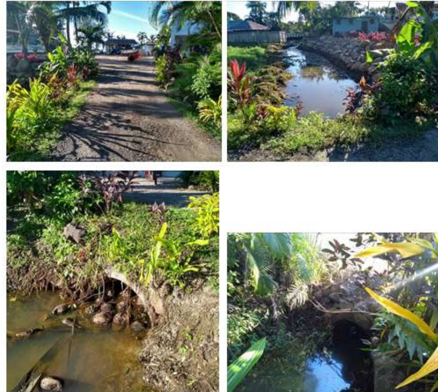
Koka Lagoon existing culvert
