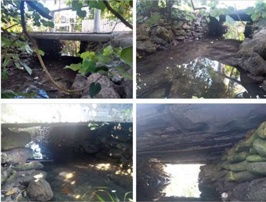
Existing Sokahala Bridge
