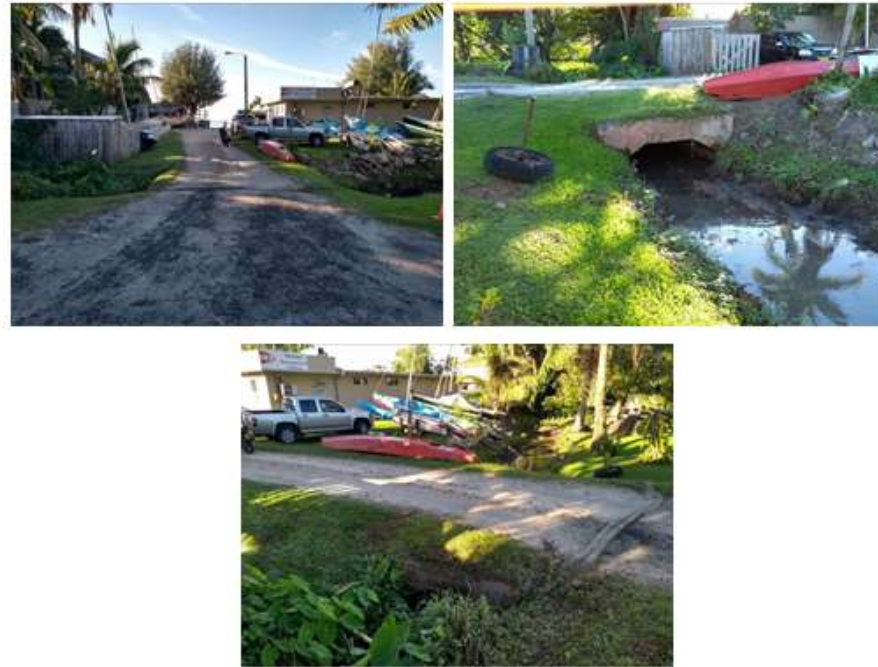
Sailing Club existing culvert
