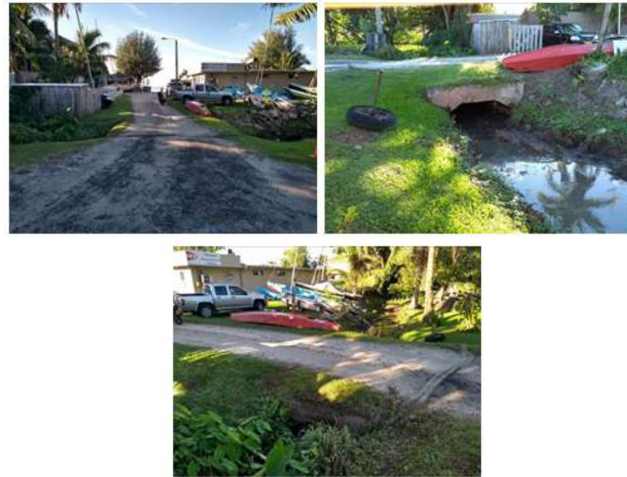
Sailing Club existing culvert
