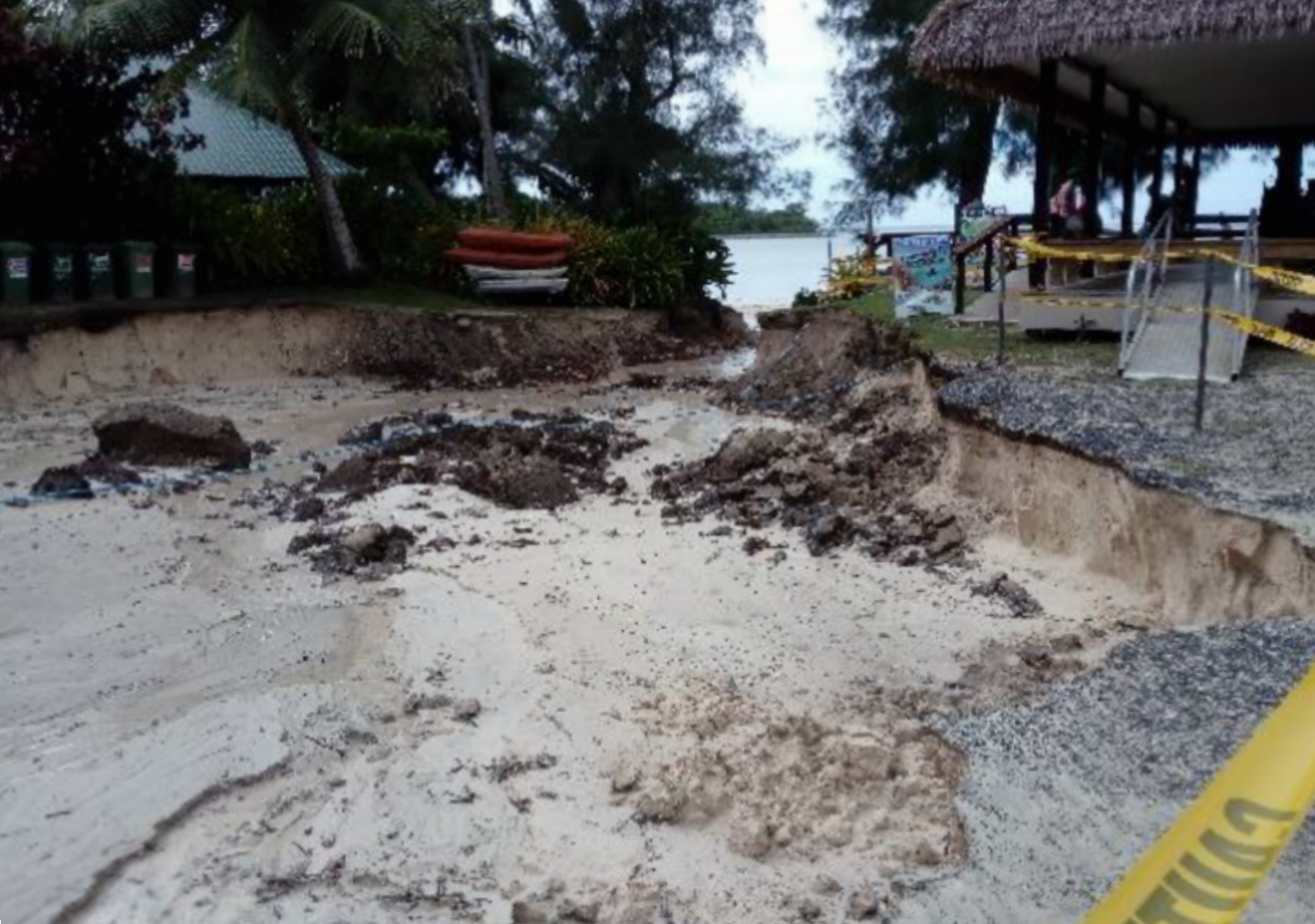
Figure 6: Erosion of land during the 2018 flooding, Muri lagoon © ICI
