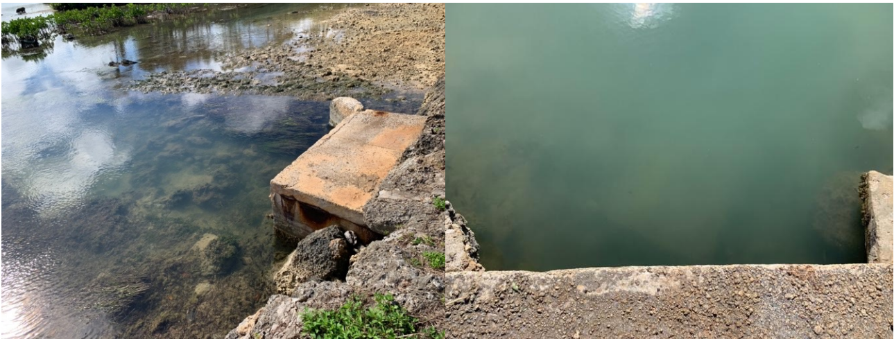
Figure 10: The two culverts in the causeway at Holeva, Hahake show the difference in water flow and quality of water. Both photos were taken on the same low tide movement with the left photo showing clear water and the second photo showing stagnant water.
