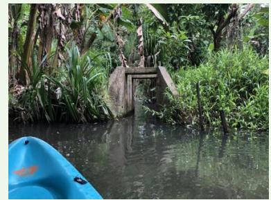
The eastern sluice viewed from inside the enclosure
