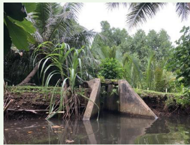
The western sluice viewed from the channel
