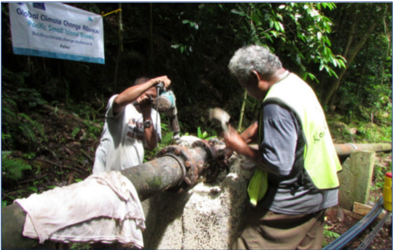
Figure 5 Pipes being fixed on an outlying Palau island
