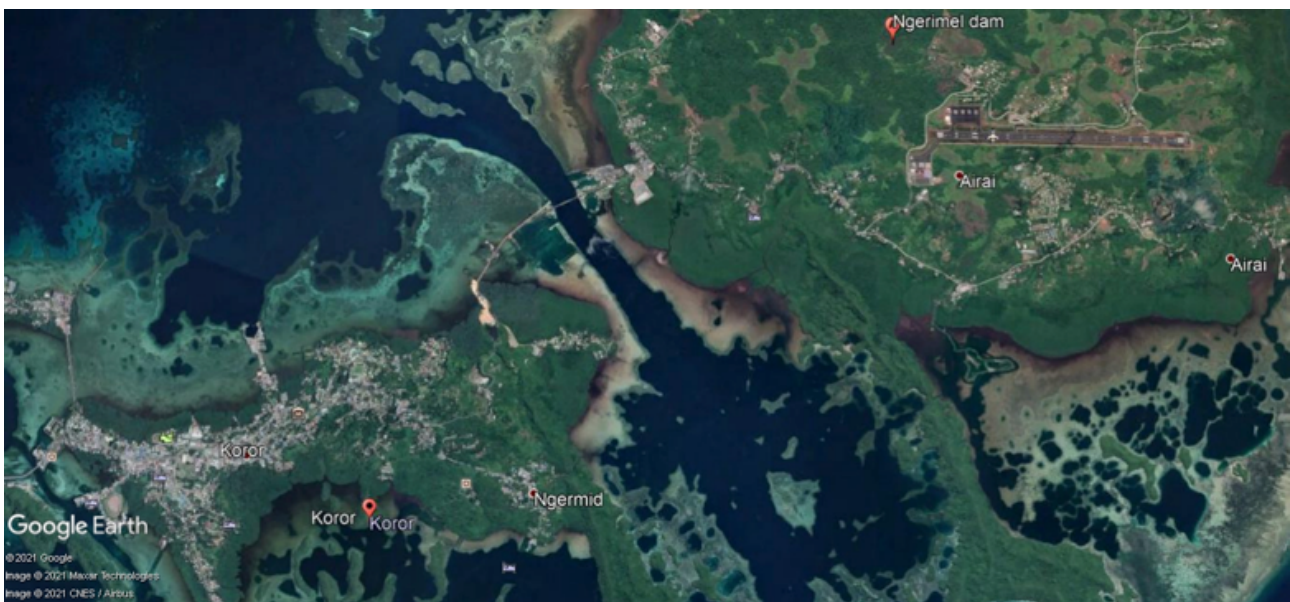
Figure 4 Ngerimel Reservoir supplying water to Koror
