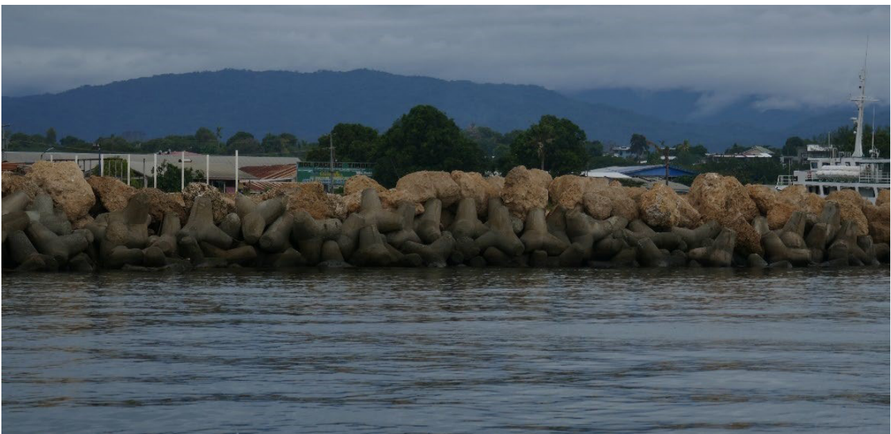
Figure 6 Seawall with Xblocs and limestone fill at Ranadi
