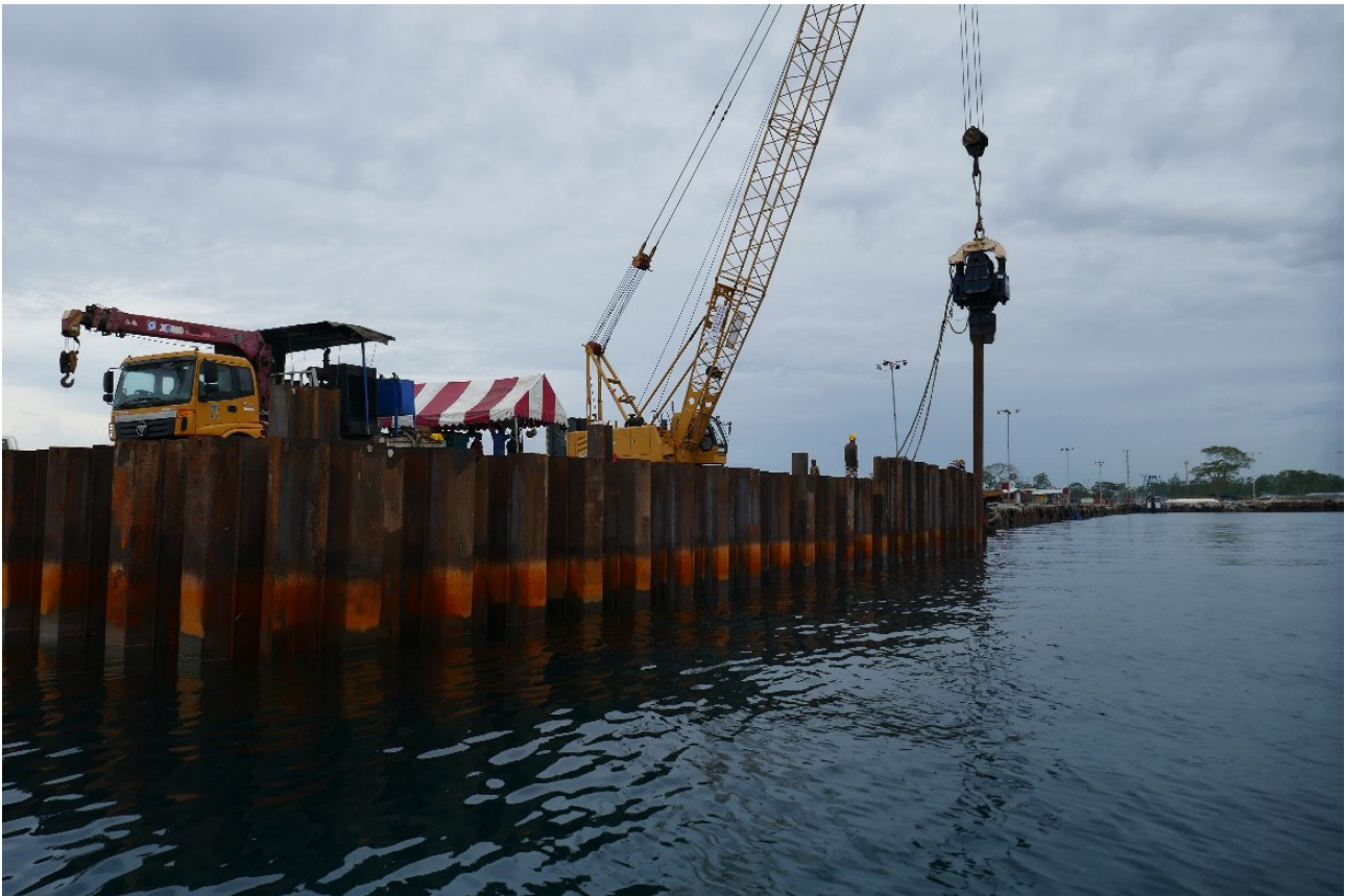
Figure 5 Wharf construction at Ranadi
