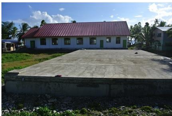
Fig 18: A water cistern for water harvesting and storage in Tuvalu. Source: http://www.sprep.org/pacc/tuvalu
