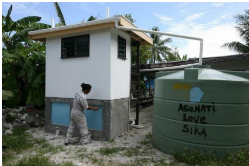
Fig 17: Water tanks from a falevatie on Funafuti Island. Source: http://www.pacific-iwrm.org/community/showthread.php?24-Photos-of-Composting-Toilets-ECOSAN-in-GEF-Pacific-IWRM-Projects
