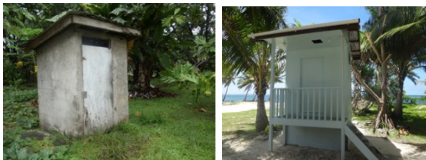
Figure 16 Comparison of the commonly used flush toilet in Laura with the waterless composting toilet demonstrated in the Laura community
