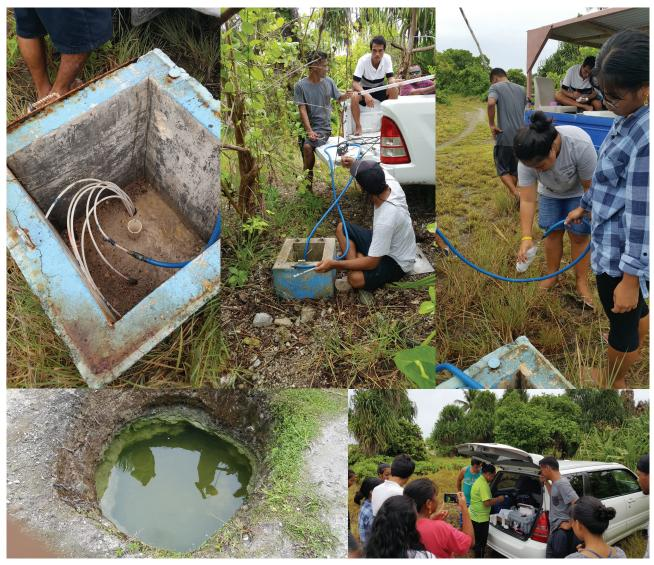
Figure 5. Showing concrete platforms of boreholes with plastic water tubes coming through concrete surface, which are used to extract water from different depths.
