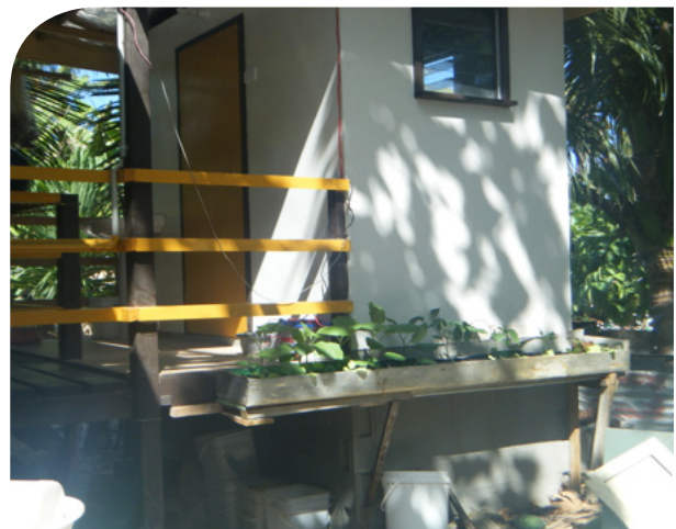
TOP RIGHT: Compost toilet construction training Finished Falevatie
