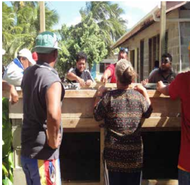
Figure 9: Eco-sanitation technical construction workshop
