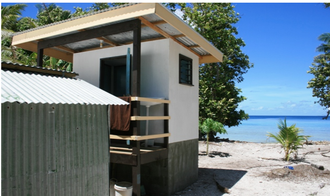
Figure 11: Composting toilet installed by the project. Prior to the installation of these toilets, waste seeped into groundwater and discharged into the lagoon
