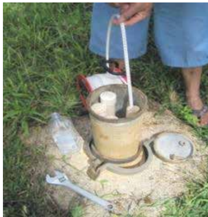
Groundwater monitoring of Neiafu Aquifer
