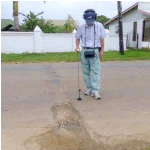
Figure 20 Leak detection in Neiafu
