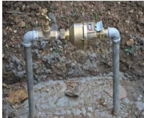
Fig 9 & 10: Meter replacement for Mbokonavera 1-5 by SIWA staff
