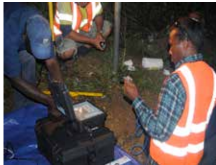
Figure 11: SIWA Staff carrying out day & night leak detection tasks
