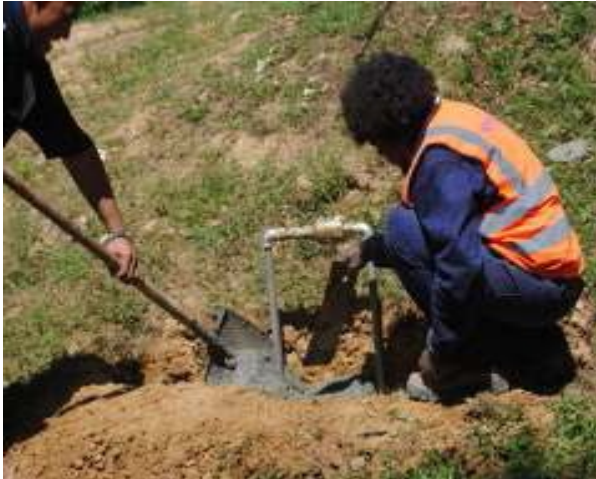
Fig 9 & 10: Meter replacement for Mbokonavera 1-5 by SIWA staff
