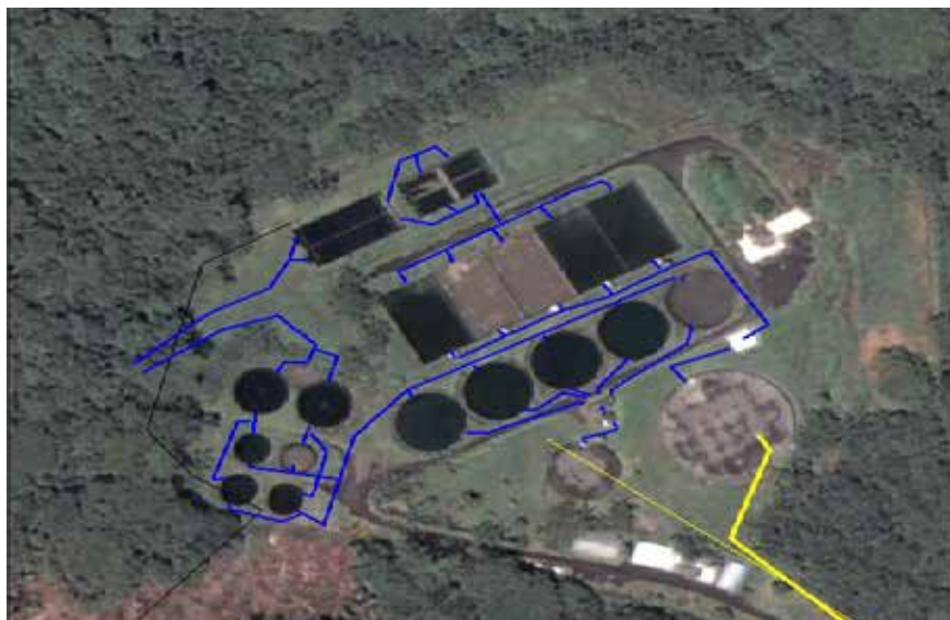
Figure 2 Aerial view of the Fuluasou Treatment Plant
