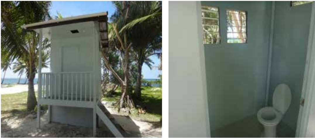
Figure 14: Recently constructed eco-san toilets as part stress reduction methods and ideal replacement for current toilets being used on Laura
