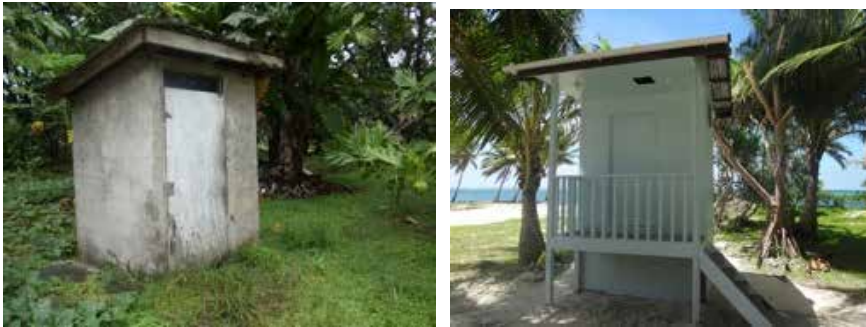
Figure 16 Comparison of the commonly used flush toilet in Laura with the waterless composting toilet demonstrated in the Laura community
