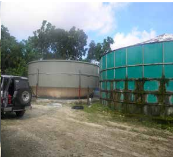
Figure 10: The new storage tanks (left) are located next to the old leaking storage (right) which had 456 kL capacity.
