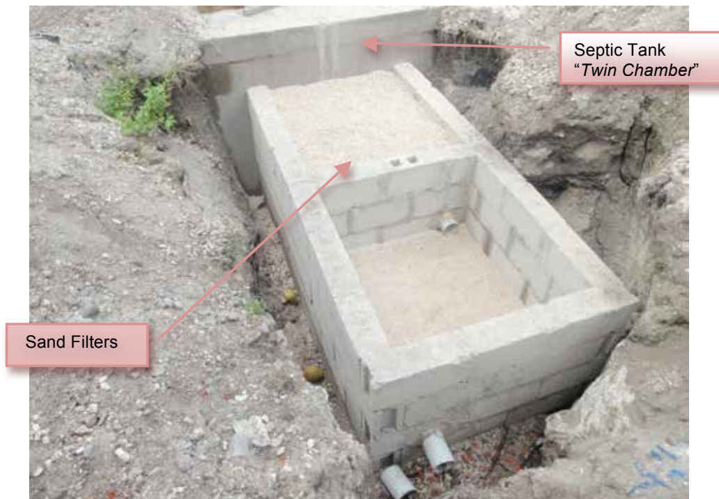
Figure 7 Prototype #1: A Conventional Septic Tank “Twin Chamber” added with two stages Sand Filters as Secondary Treatment to improve the waste water effluent prior being discharge via irrigation.
